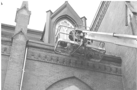
**NEVER FINISHED...** Or at least, so it seems, with the downspout and gutter at the ramp entrance. Ice build-up and melting over the years has affected the plaster on the inside by the window, and previous attempts to control ice and melting have not worked. Last week, workers installed a heavier gauge seamless downspout, soldered the joints, and placed a heated electric coil into the downspout, gutter, and along the roof edge to prevent ice formation. Let's hope this works!
