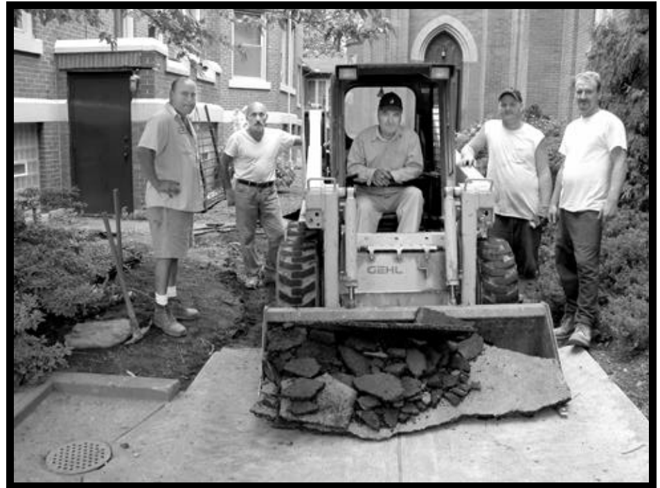
CECCHI CONCRETE CO. is donating all the concrete work for the walks in the garden area between the rectory and the church. The crew first had to dig up and remove all the old concrete and asphalt. Then Joe Calamante set the forms for the concrete which was poured and finished by the Cecchi Co. Pictured above from left to right are Rick Cecchi, Mark Cecchi, Lou Cecchi (sitting in the bobcat tractor and owner of the company) Keith Brown and Mark Gannon. Lou Cecchi is a member of the parish and graciously offered his assistance when he found out we needed this work to be done!
