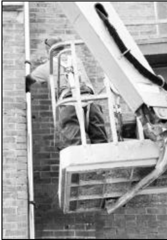
Workers used a crane to reach the top of the downspout while replacing it.
