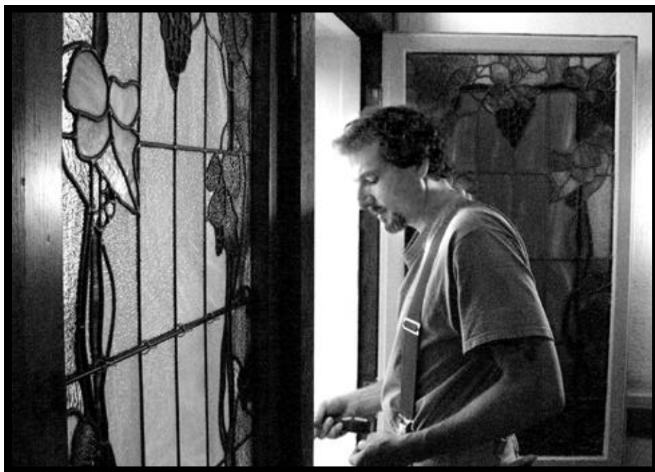
Getting Closer to Completion! A carpenter installs the restored stained glass windows in the stairwell to the Rectory's second floor.
